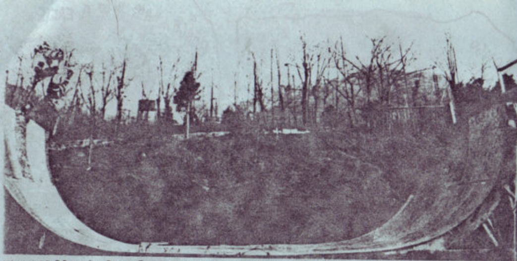
VISION OF RATONES RAMP II: 2.4 MT. OF HIGH, 3.4 MT. WIDE WITH 3.5 MT. OF FLAT BOTTOM INVERT: ECCO LA RAMPA DI GENOVA
